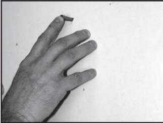
4. Press 4 appropriately sized sheetrock anchors into the wall so that the sheetrock anchor is flush with the wall.
