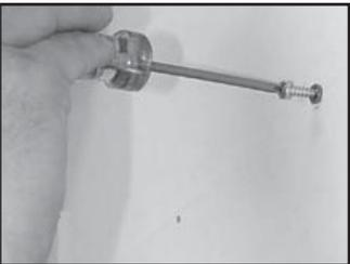
5. Screw four #8 flathead wood screws (1 inch or 2.54 cm) into the wall anchors. Make sure you leave 1/4 of an inch (0.635 cm) between the wall and the head of the screw.
