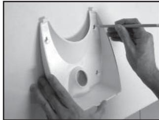
2. Using the repositional base as a guide, mark the 4 wall holes with a pencil or pen.
